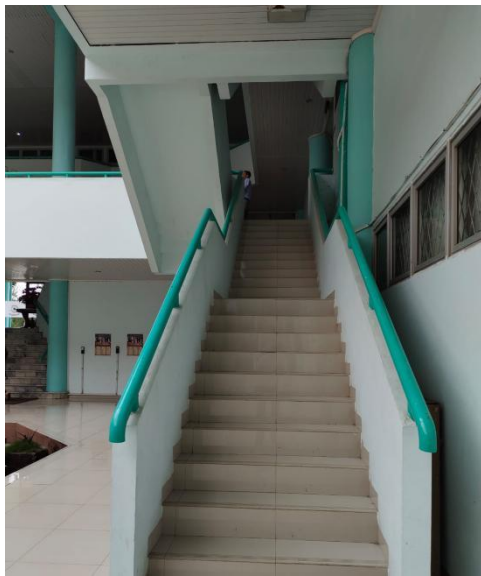
Figure 1. Accessible stair handrail.
